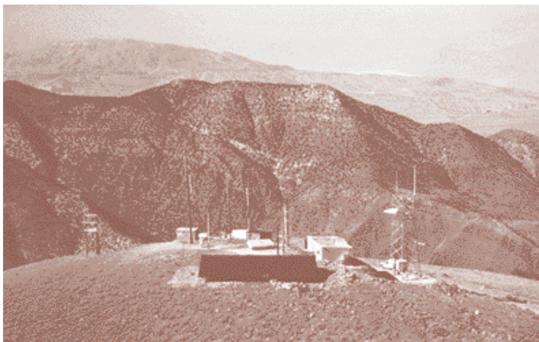
Communication site powered by solar with LP Gas back up.
