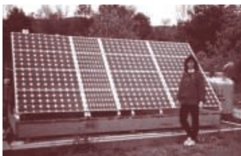
A solar photovoltaic array / LP Gas hybrid. LP Gas tank shown in background.
